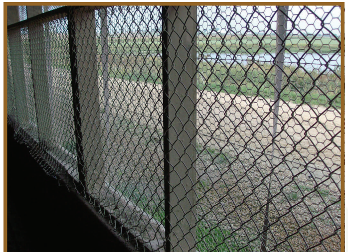
PVC coated hex wire anchored on the barn
